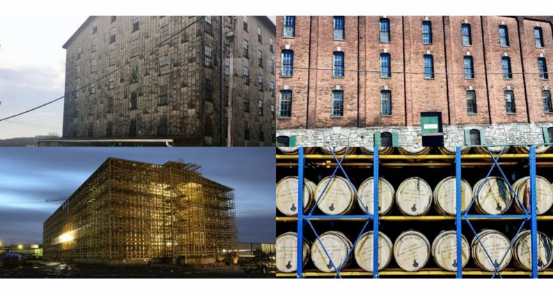
Traditionally, these structures would all be constructed from an oak interior (or skeleton) and sheeted with iron. These colloquially have been referred to as Ironside Rickhouse. Today, brick, cement and even more modern palletised warehouses have been used.
